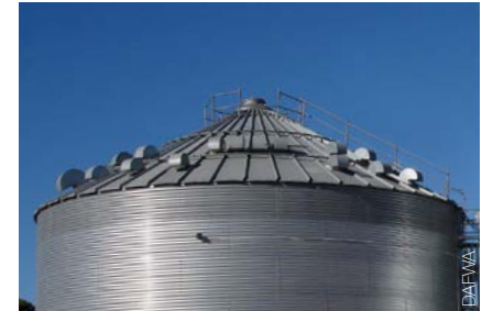
Silos with ventilation units
